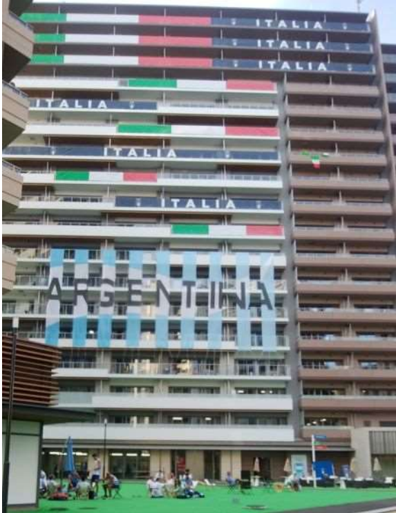
The national frags are affixed to the wall
